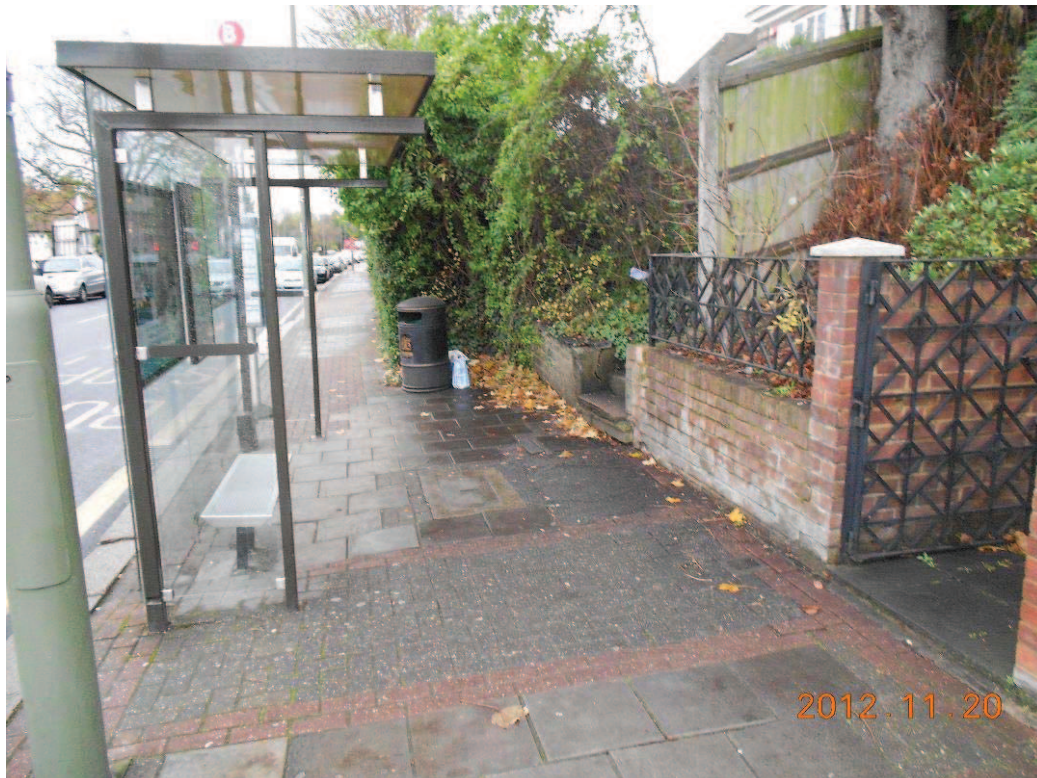
Bus stop Finchley Road with start of steps just visible.
